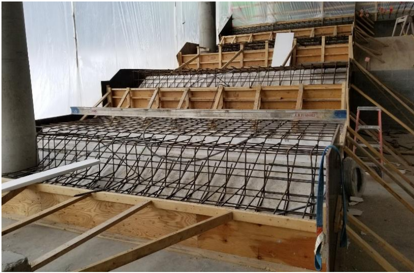
Left: The social stair is all ready to be poured on Monday as the rebar and the outlet boxes are installed. Above is a photo of the wall framing and duct work on the third floor. Left is a drone view of the front of the school and the completed sheathing.
