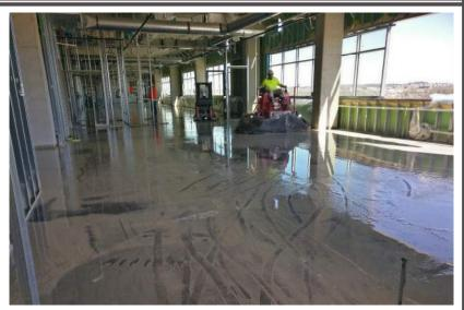
We have started finish flooring on the third floor! Above you can see riding machines polishing the concrete floors, leaving a wet surly on the floor that is cleaned up after the polishing is complete. Below: Brick has continued with the Carbon Black brick that is aligned in a stacked bond shown below.
