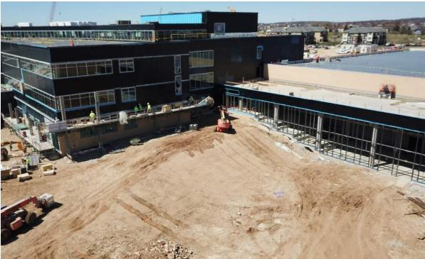
Left: Work on the brick continues around the school as the south side of the fieldhouse is complete above, we move on to wrapping around the south side of the school. In addition this photo shows the curtain wall framing for the windows at the social stair location at the Fieldhouse. Lower Left: Slab on Grade continues on site with the ground thawing. Final photo is of the borrow lites that are being installed in the Atrium.
